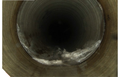
Psn. 5 - 7; Crack formation, Surface crack, longitudinal, Width = 223mm
